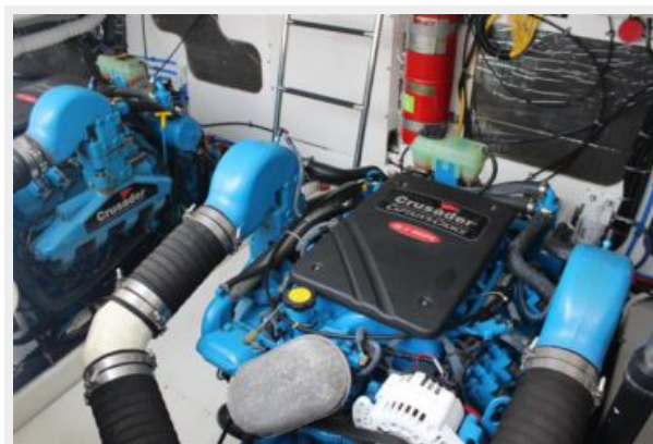
36 Tiara Sovran Engine Room
