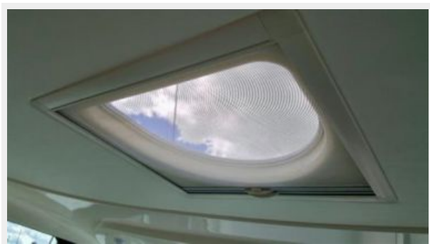
Skylight at Helm
