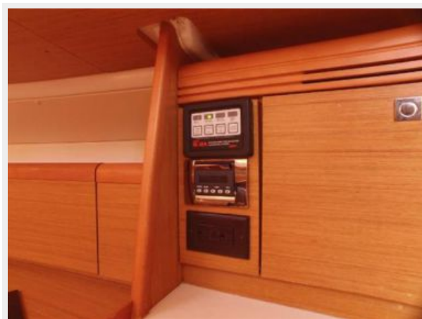
Galley A/C Control and Propane Control
