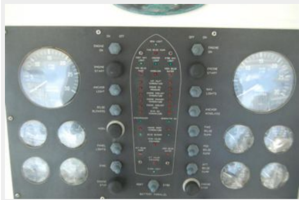
Helm Control Panel.JPG
