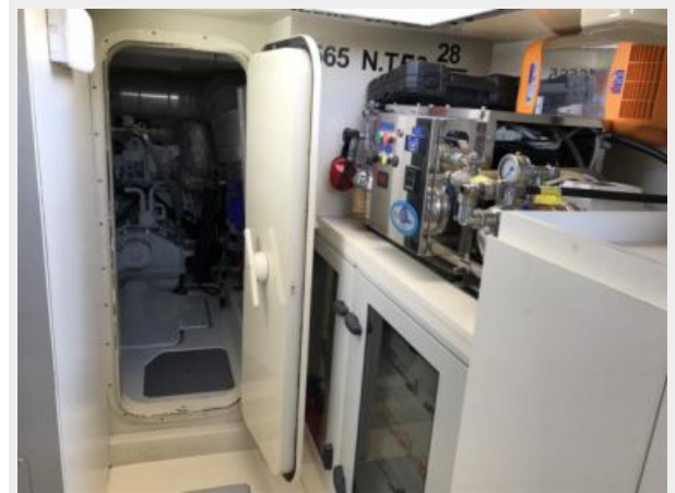
Engine Room Door
