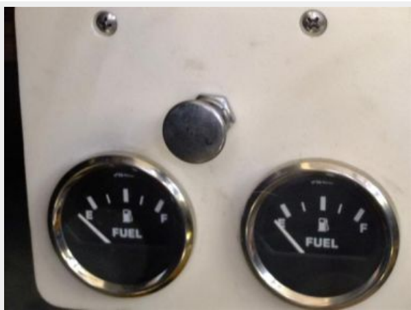
Grand Banks 42 - Engine Room Fuel Gauges
