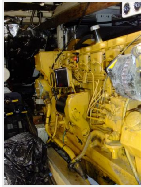
Grand Banks 42 - Engine Room STBD Engine
