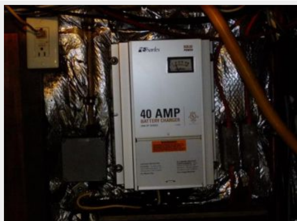
Grand Banks 43 - Engine Room Battery Charger
