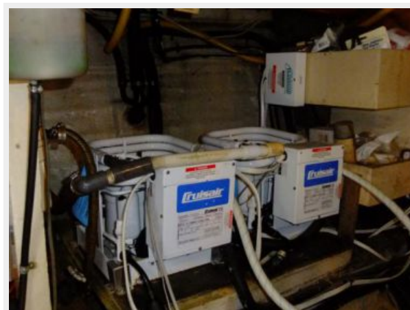
Grand Banks 42 - Engine Room A-C Systems
