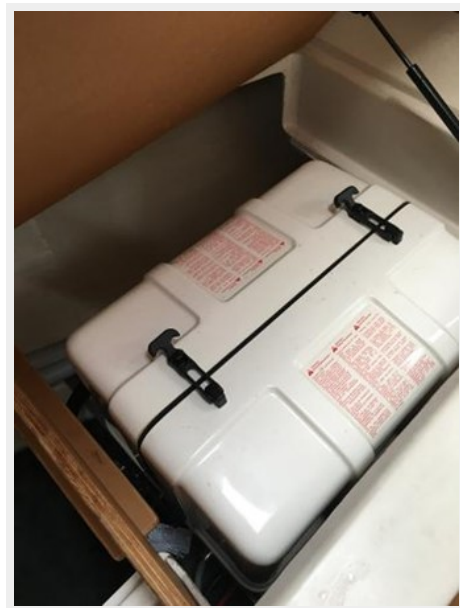
2004 Catalina 470 - Fischer panda generator
