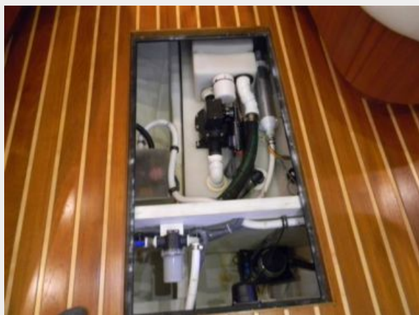
Cabin bilge access
