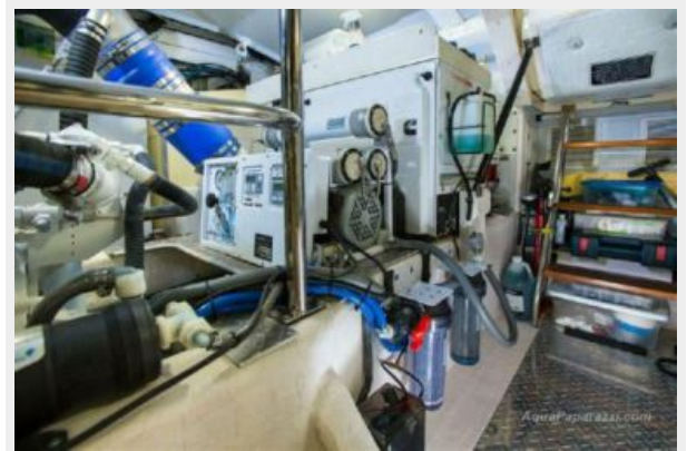
52 Sabre Engine Room
