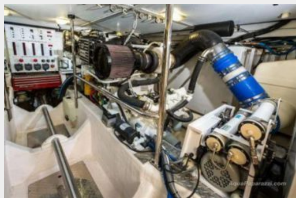
52 Sabre Engine Room
