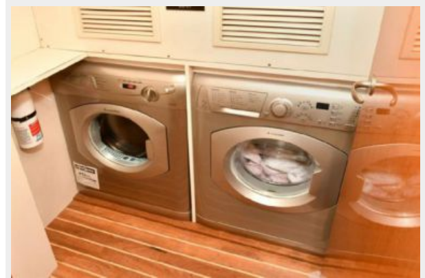
Washer/ Dryer Units
