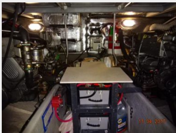
Moondance engine room aft 11-4-17
