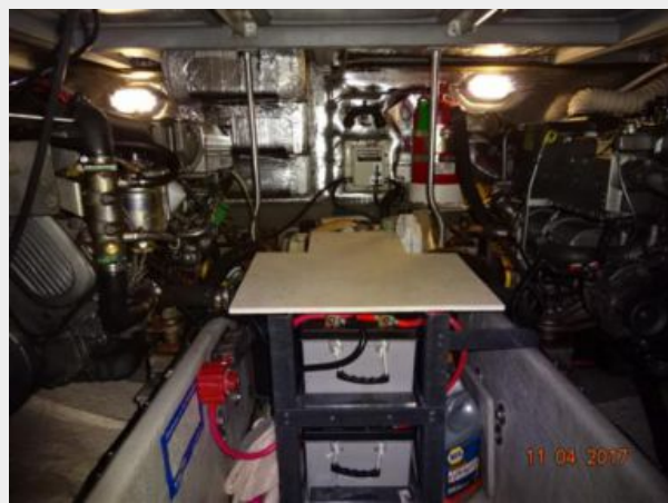
Moondance engine room aft 11-4-17
