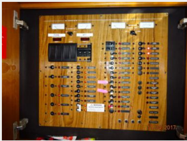
Moondance electrical panel 11-4-17
