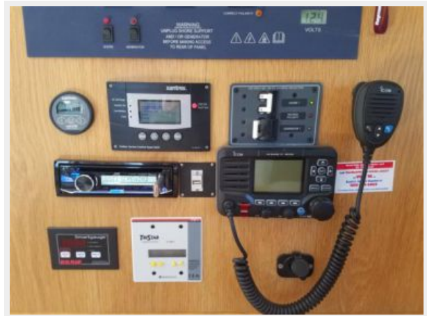
Broadblue 435ST instrument control panels
