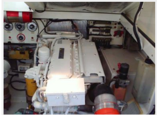
Engine & Mechanical Equipment 5 - Starboard Engine
