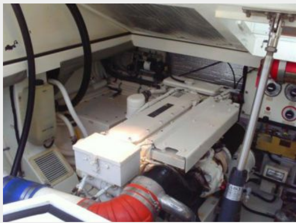
Engine & Mechanical Equipment 4 - Port Engine
