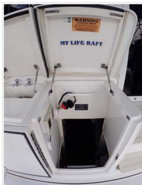
Engine Room Entry
