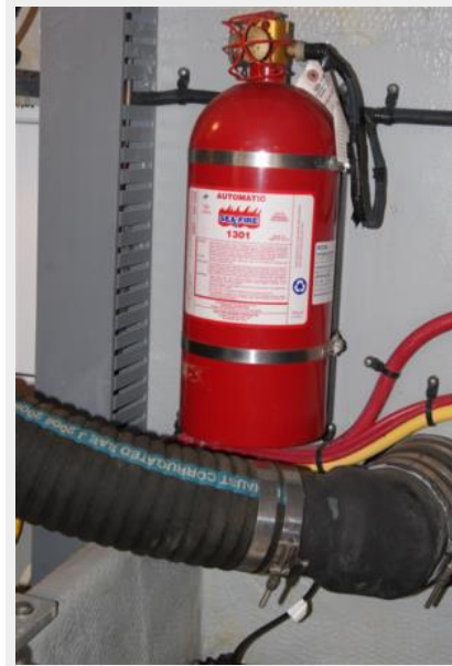
321 Engine Room Fire Extinguisher
