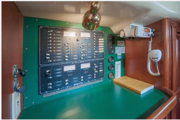
Nav. Station Primary Elec Panel
