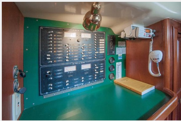
Nav. Station Primary Elec Panel
