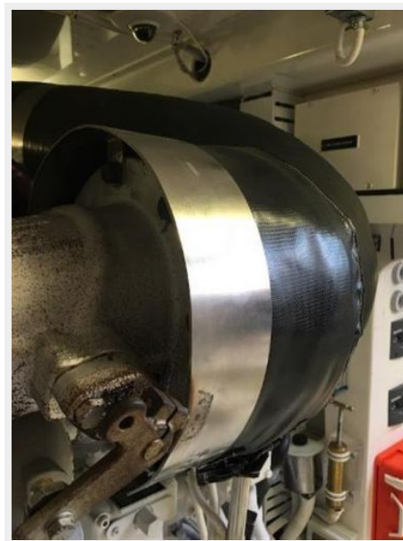
Upgraded Exhaust Vibration Isolator
