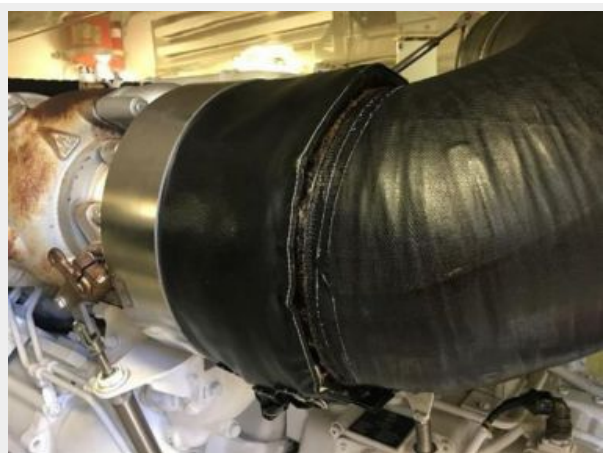
Upgraded Exhaust Vibration Isolator
