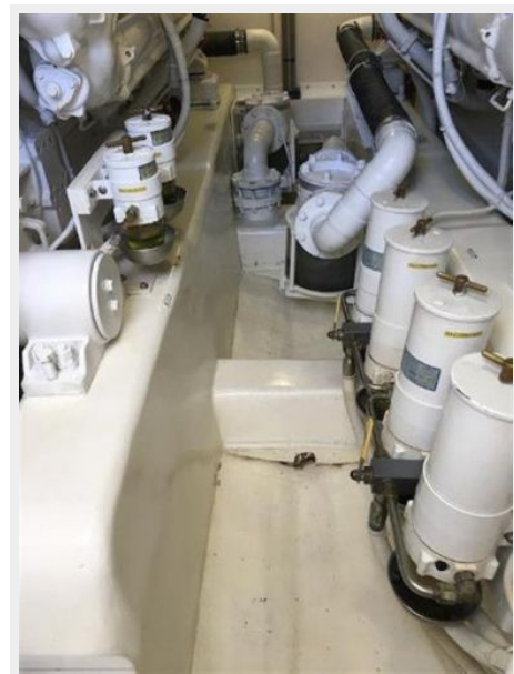
Dry Bilge Detail
