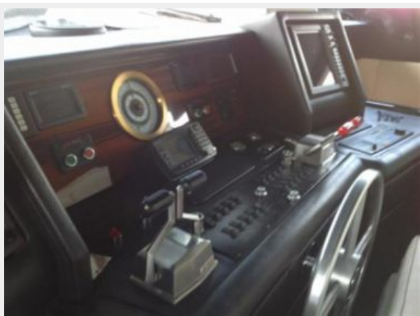
PILOT HOUSE - New Electronics in Progress
