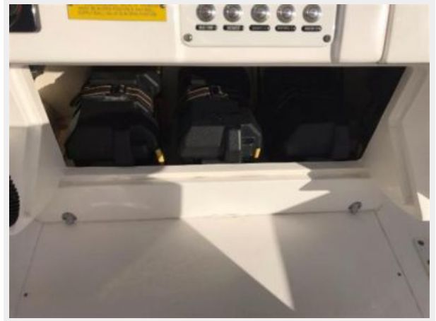
327 Intrepid | Battery Boxes
