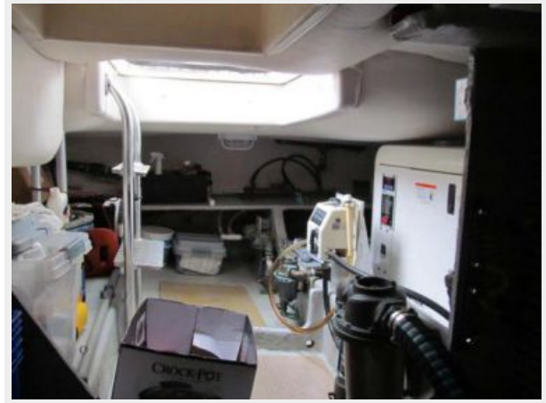
Engine Room Aft
