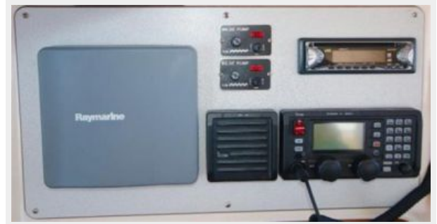
Electronics at Nav Station
