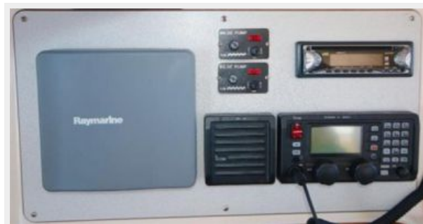
Electronics at Nav Station
