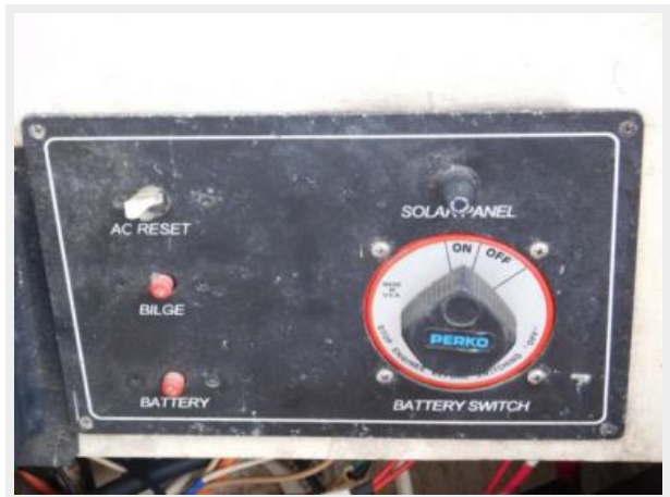
Solar Panel Power Switch
