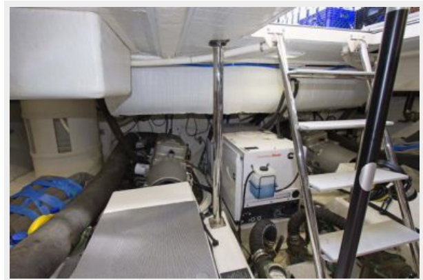
Engine Room Aft
