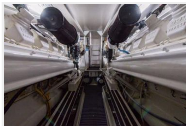
Engine & Mechanical Equipment 8
