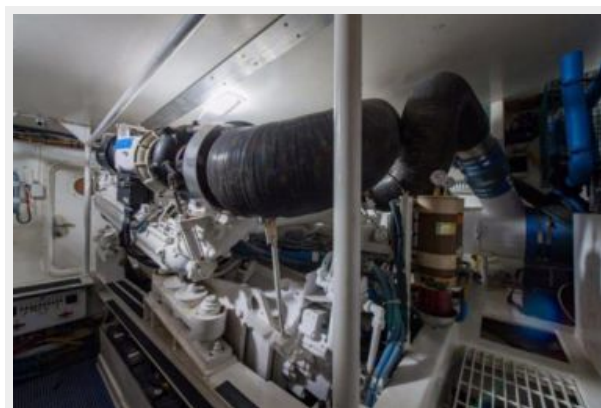
Engine & Mechanical Equipment 6
