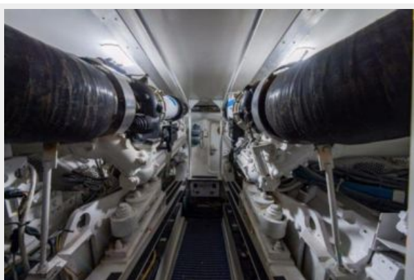
Engine & Mechanical Equipment 1
