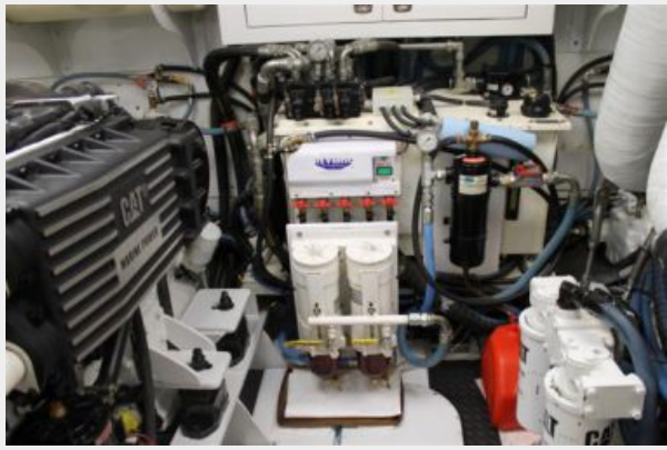
Engine Room Looking Aft
