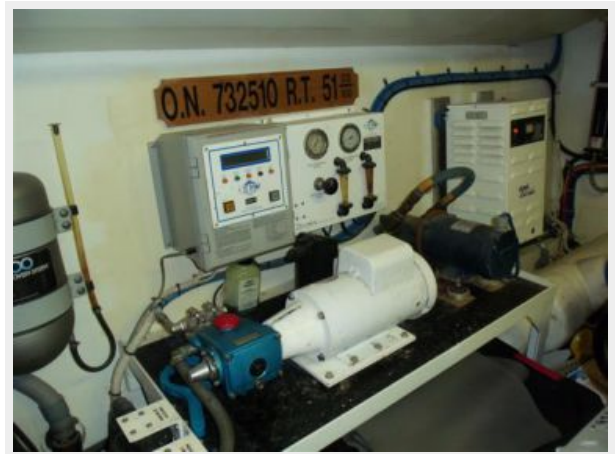
Outboard Starboard Engine
