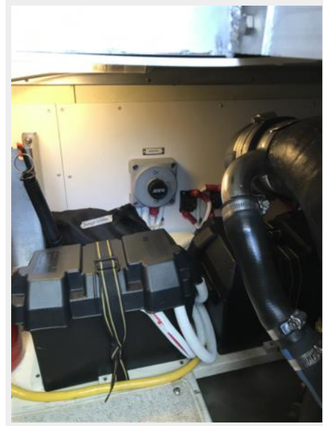
360 Carver SS - Engine Room
