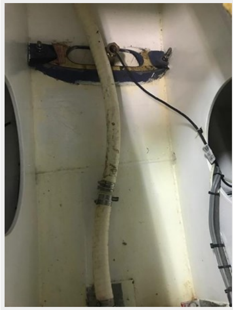
Spaces Under Crew Floor 2
