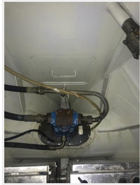
Spaces Under Crew Floor 3
