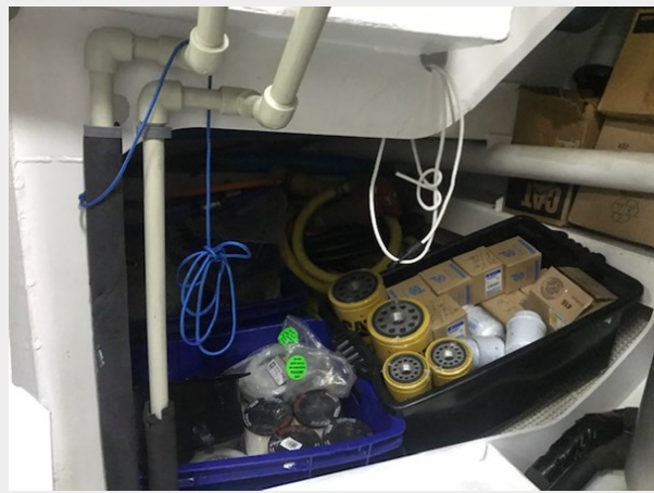
Lazarette bidge under floor plates 4
