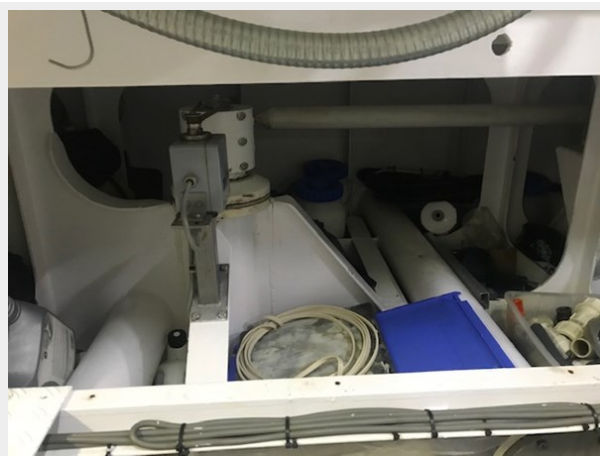
Lazarette bildge under floor plates 2
