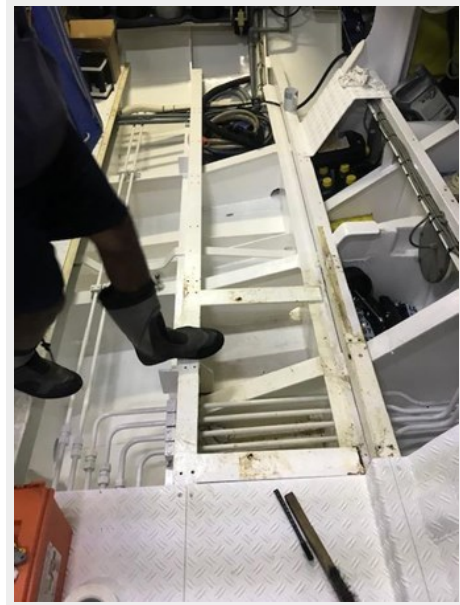
Lazarette bidge under floor plates 5
