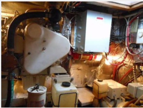
Engine Room looking aft to port
