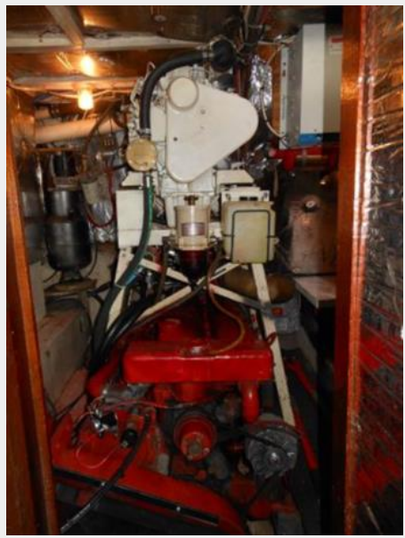
Generator above main engine
