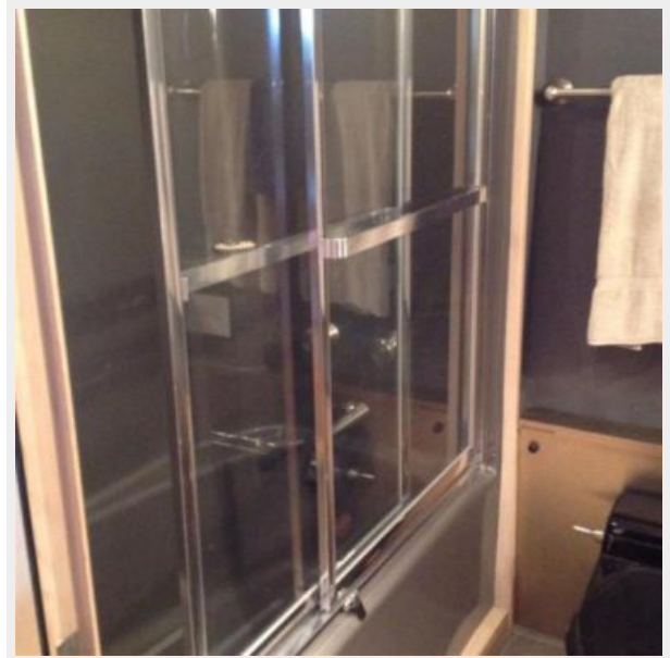
STARBOARD GUEST HEAD - Shower w/Sliding Glass Enclosure
