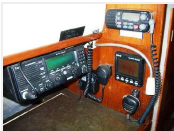
Nav Station Electronics
