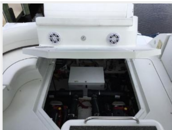
Engine Room Access
