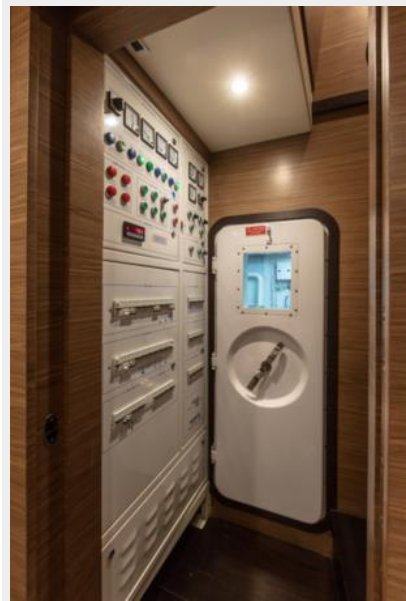
Entrance to the engine room
