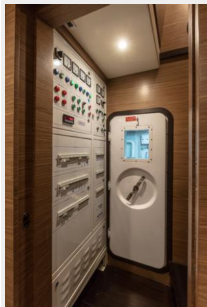
Entrance to the engine room
