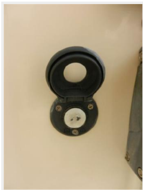
Electric winch control
