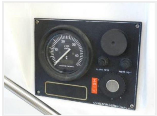
Engine panels in cockpit
