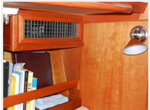
Air Conditioning vent in salon
