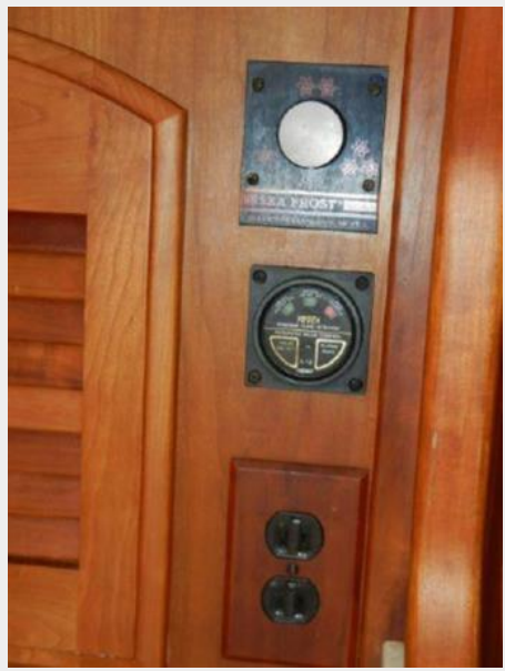
SeaFrost control, propane detector
