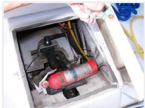
Access to Steering & Rudder Post
