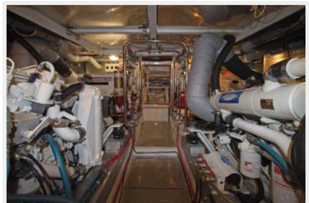
Engine Room Aft
