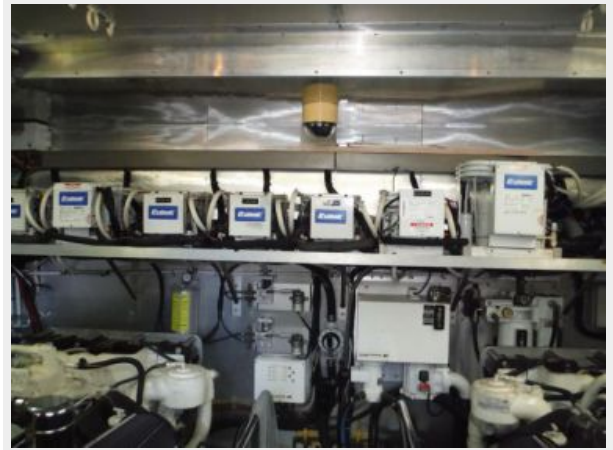
Engine Room Forward
