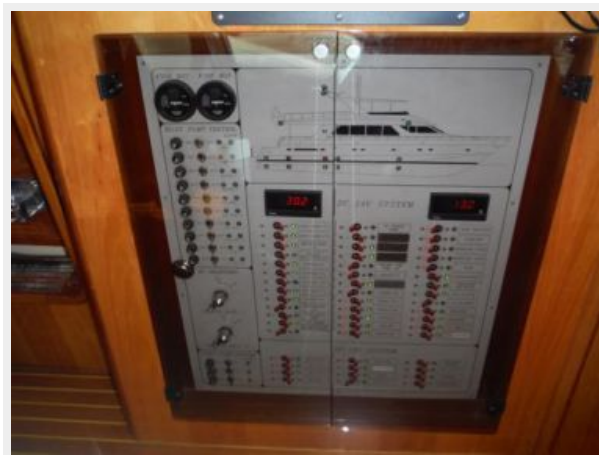
Pilothouse DC panel
