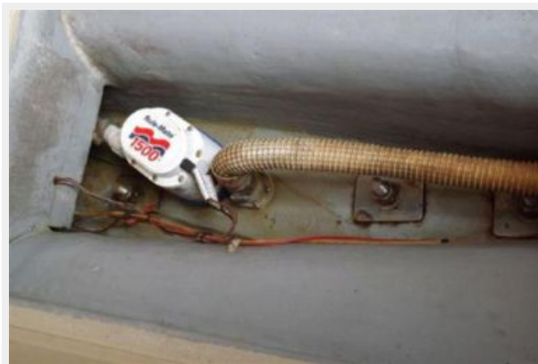
New Bilge Pump
